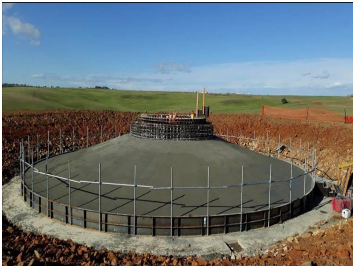
Figure 3.5: Typical Turbine Foundation
