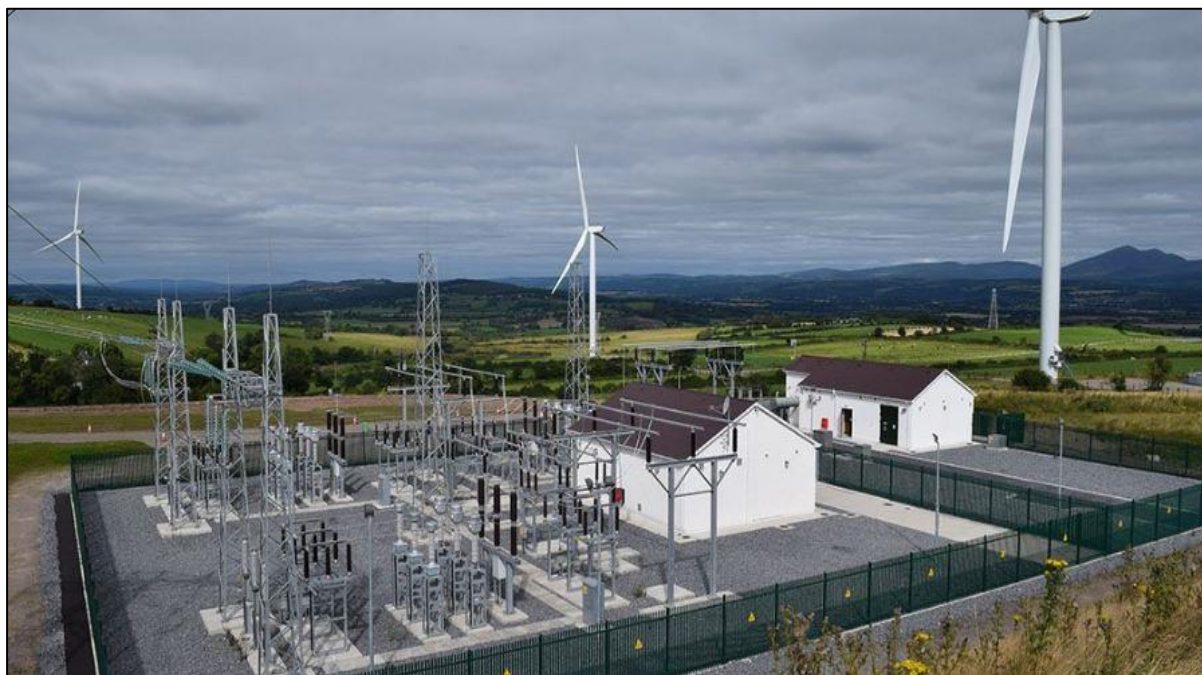
Figure 3.6: Typical 110kV AIS Substation
