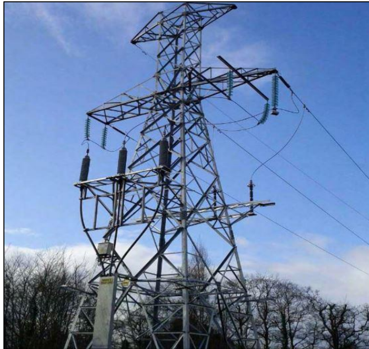
Figure 3.9: Typical End Mast
