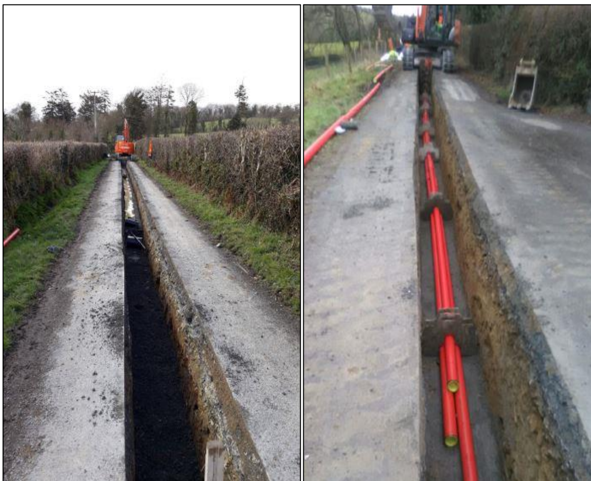
Plates 1 & 2: Typical Trench Construction
