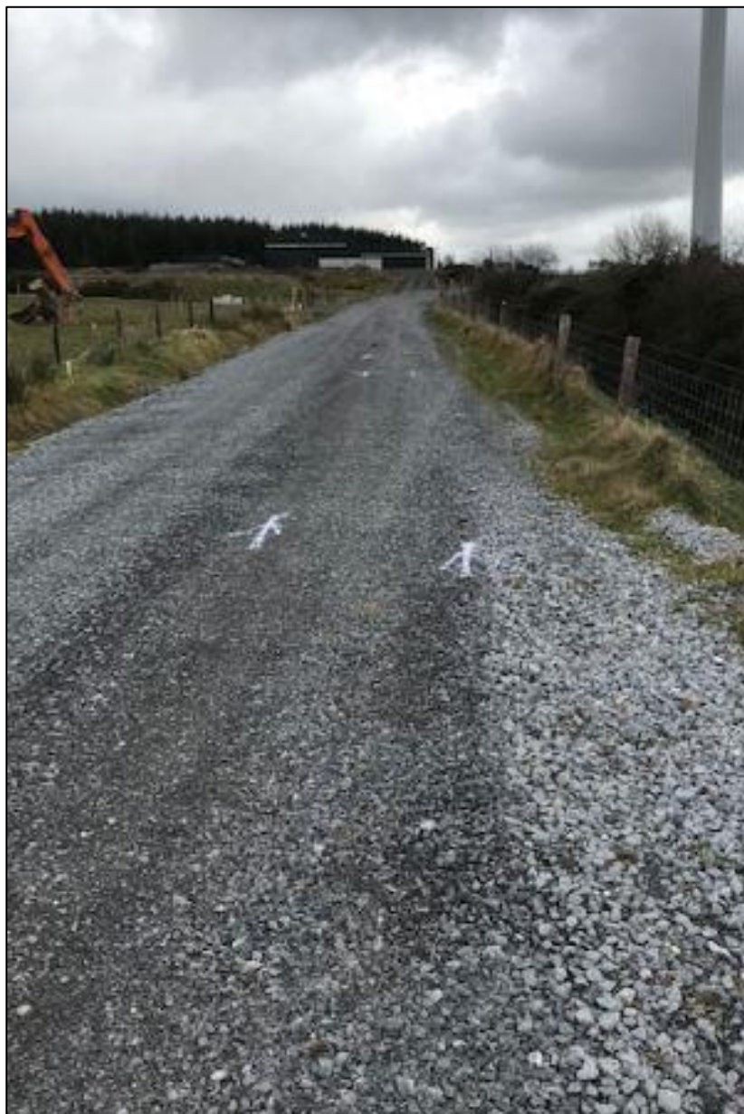
Figure 3.7: Typical Access Track
